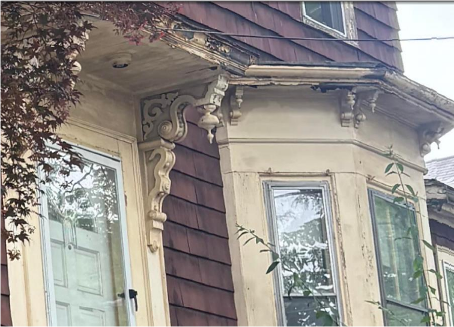
Above: Details of front entrance and bay window Italianate brackets on 83 Wallace St
