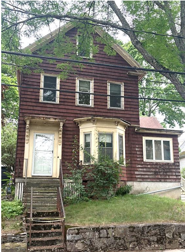
Above: Front elevation of 83 Wallace St
