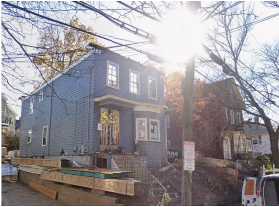
Above: 85 Wallace St (Italianate home being demolished next door)
