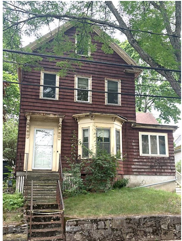
Above: Front elevation of 83 Wallace St
