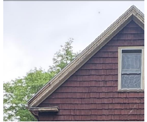
Above: Details of rear boxed cornice on 83 Wallace St
