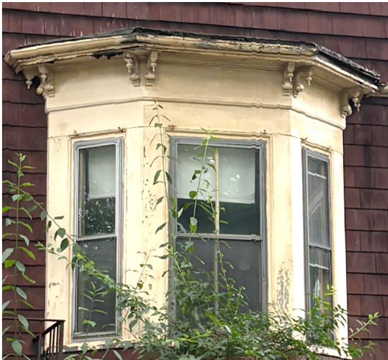
Above: Details of projecting bay window with Italianate brackets on 83 Wallace St
